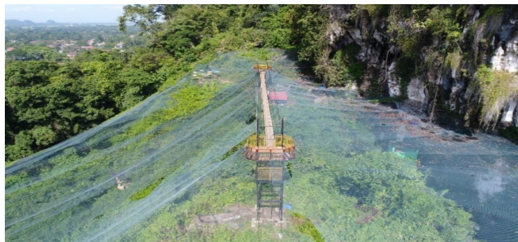
Fig. 4. The panorama of Helena sky bridge view from above
